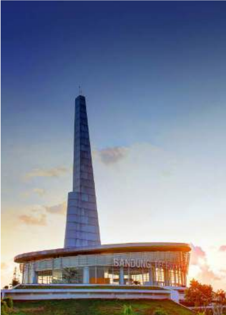
Bandung Techno Park (Sumber: Telkom Foundation)
